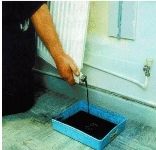
Accumulation of sludge is an indication of corrosion in the heating system and may be accompanied by the accumulation of gases within the radiators – which may be mistaken for air accumulation in very severe cases.
